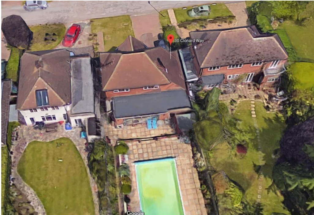
Google image- rear elevations
